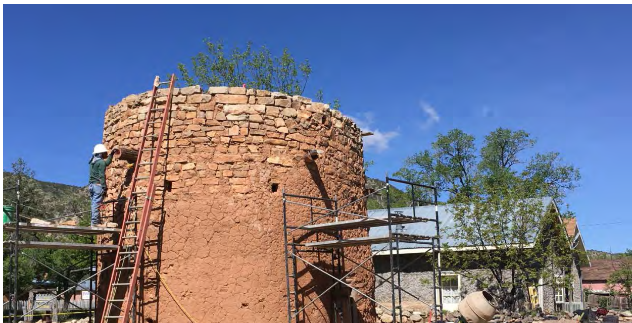
Torreón at Lincoln Historic Site under construction
