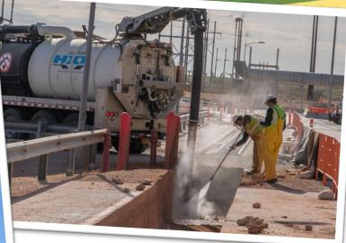
Multiple hydro-excavations are happening at WIPP for new air, fire water and fiber optic lines.
