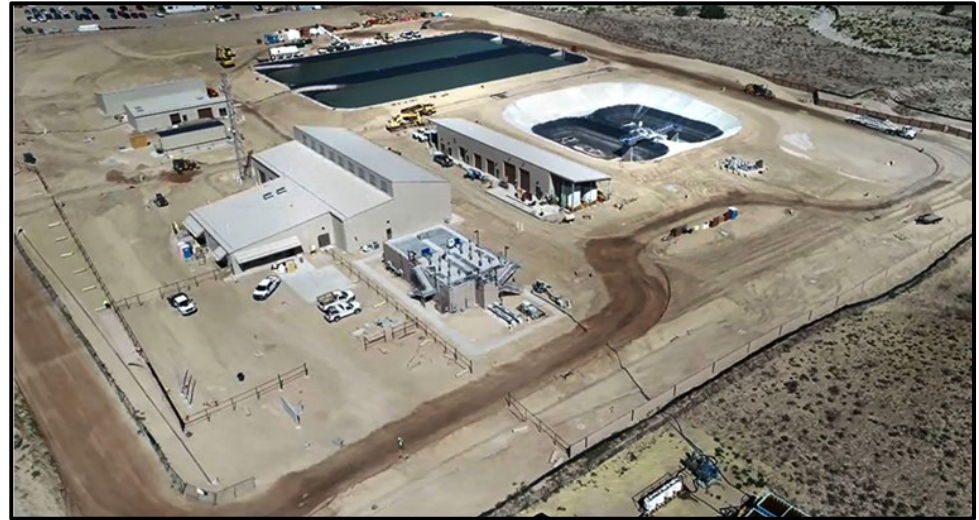
Cutter Lateral Water Treatment Plant
