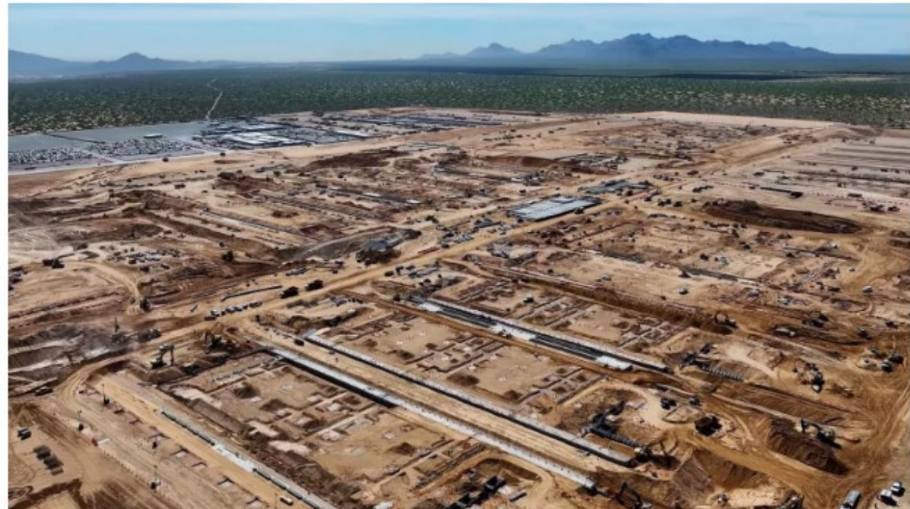
The building site for the Project Jupiter data center in Doña Ana County, New Mexico
