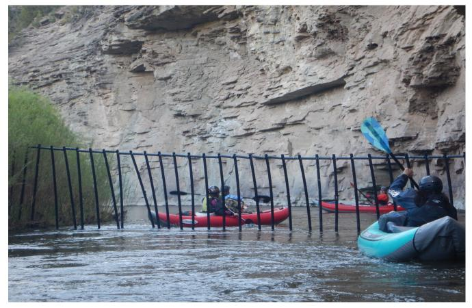
Hanging PVC pipe that swings allowing both watercraft and debris to pass through.
