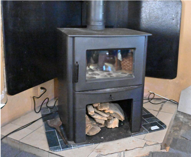
New EPA-certified high-efficiency wood stove installed in Robert Allen's home
