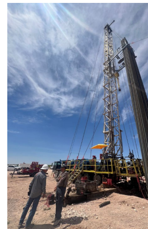
Figure 3. Modern Plugging Rig
