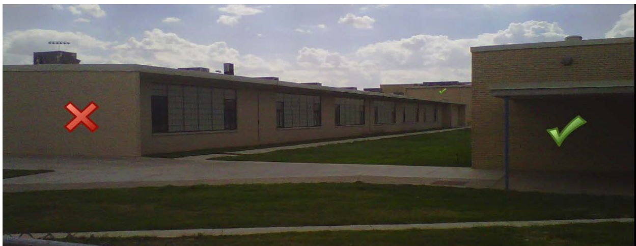
Photo 1. Lovington’s Freshman Academy (marked with a red X) sits adjacent to two Lovington High School Buildings (marked with green checkmarks).
