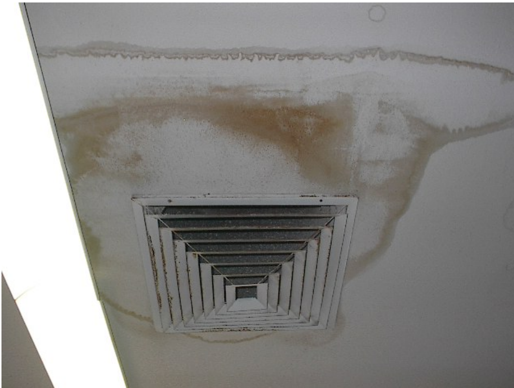
Figure 20. Excessive water damage to ceiling near ventilation system.
