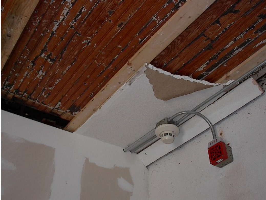
Figure 20. Excessive water damage to ceiling near ventilation system.
