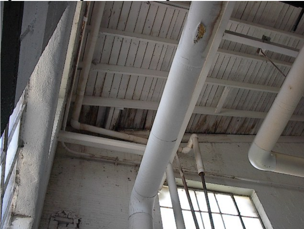
Figure 4. Water damage to boiler room ceiling and walls.
