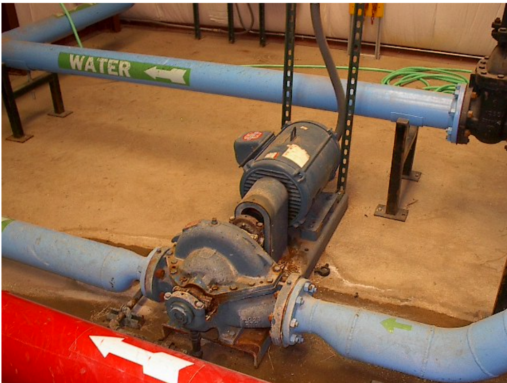
Figure 12. Rust corrosion to water softener system.
