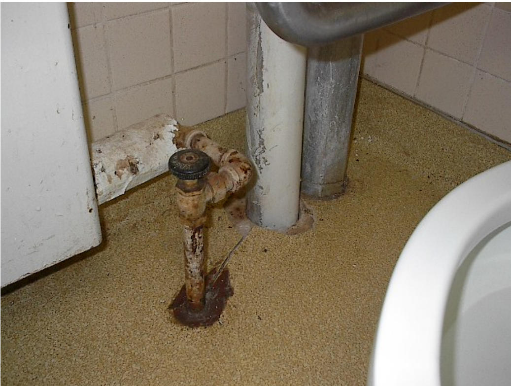
Figure 14. Partially insulated, rusty hot water valve in resident common area.
