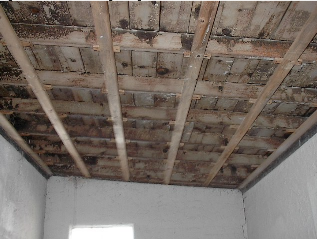
Figure 22. Warehouse wall and floor damaged by heavy rains.
