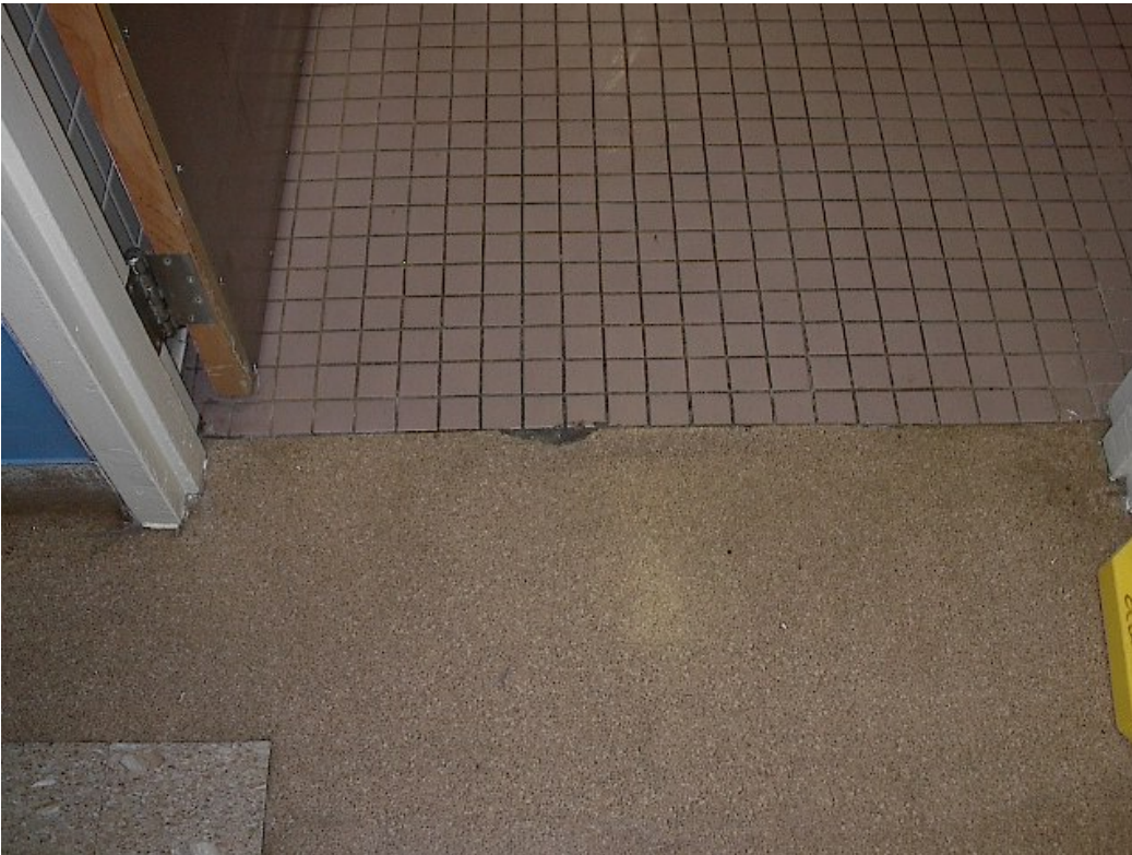
Figure 8. Jagged threshold edge exposed to residents.
