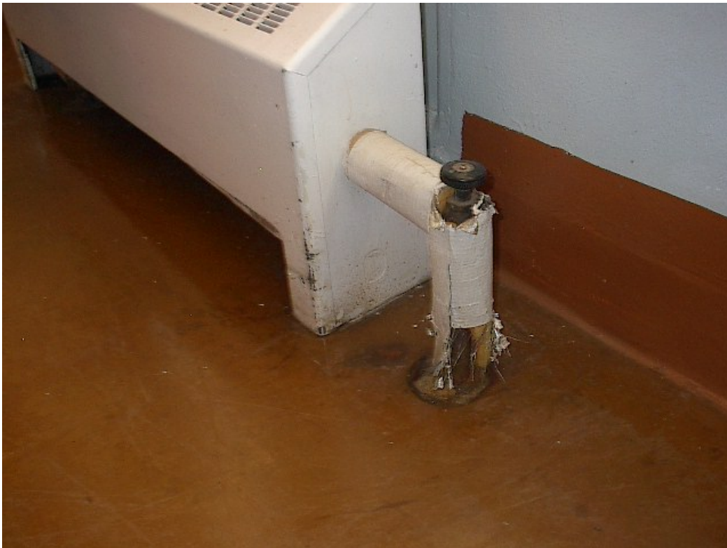
Figure 10. Partially exposed hot water valve.
