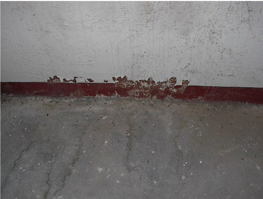
Figure 22. Warehouse wall and floor damaged by heavy rains.
