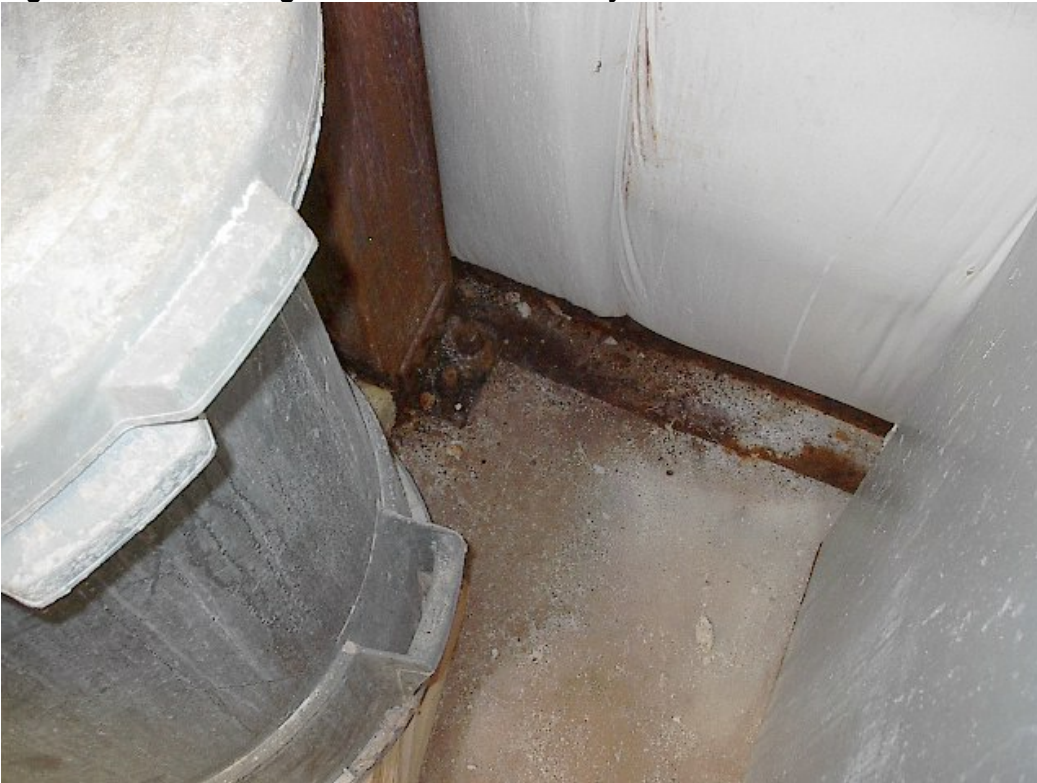
Figure 14. Partially insulated, rusty hot water valve in resident common area.
