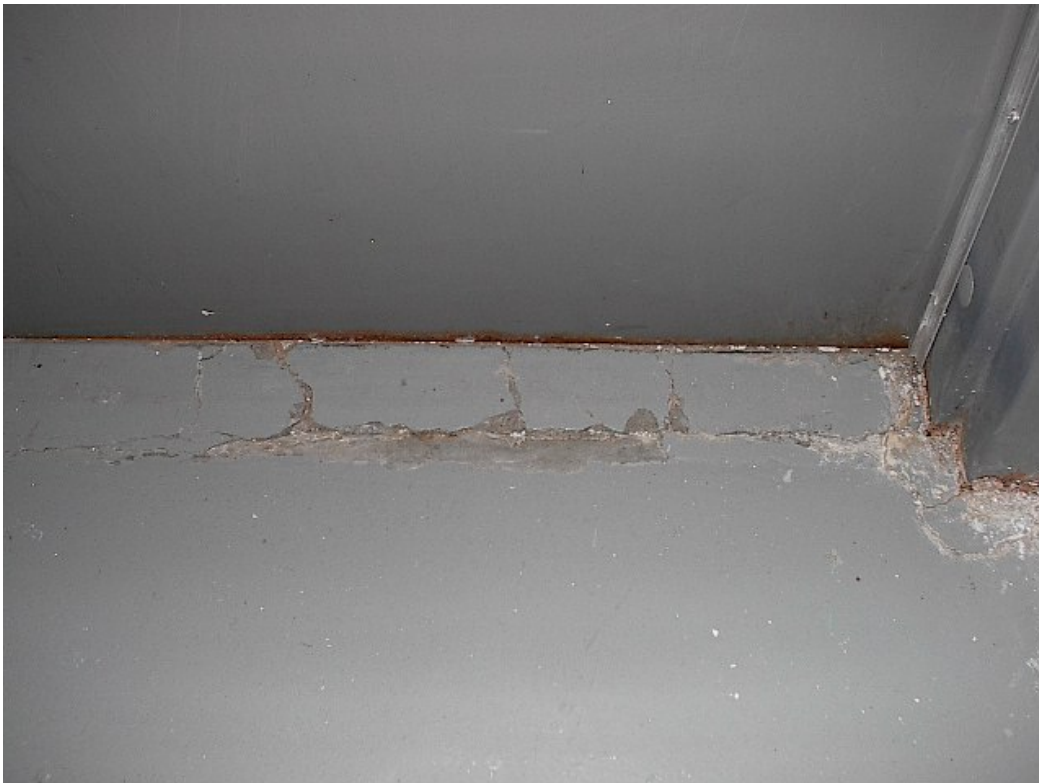
Figure 6. Jagged floor edges exposed to residents
