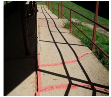
NMBHI Cracked Sidewalks
