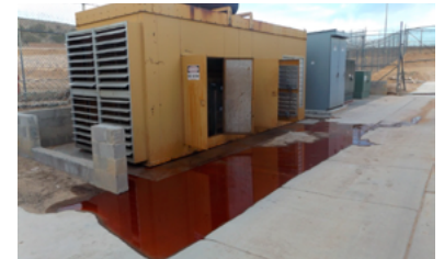
Failing Generator with Pooling Coolant
