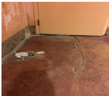
National Hispanic Cultural Center Sinking and Cracking Floors
