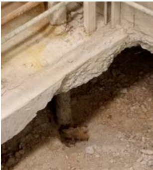
Drain Rot and Settlement at NMDA
