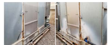
Corroded and Leaking Chiller at National Hispanic Cultural Center
