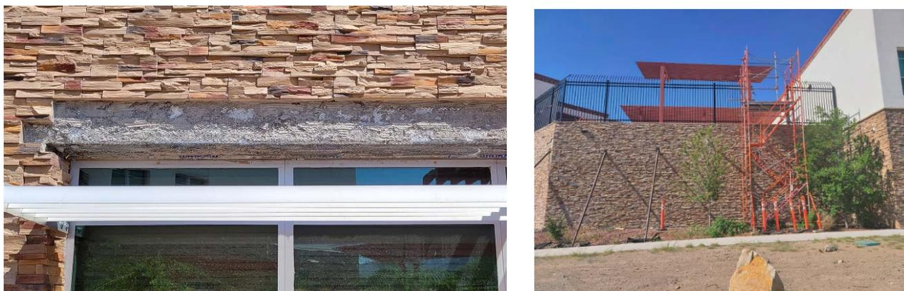
Left: Exterior trim above windows failed to properly adhere. Right: Work to repair damaged retaining wall.
