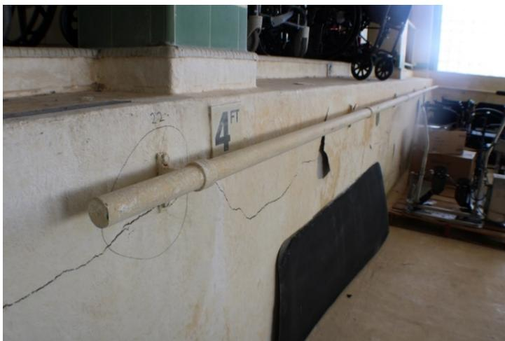
Cracks in unused therapy pool used as wheelchair storage.
