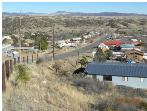
One of the residential streets that will receive a new municipal sewer line.
