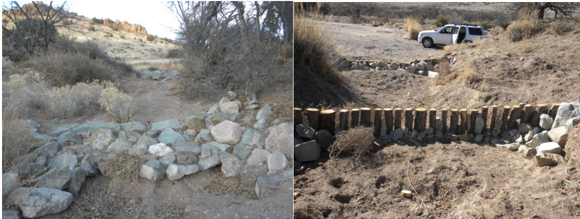
Examples of rock and wooden structures to be used to trap sediments and minimize erosion while increasing recharge to the water table.
