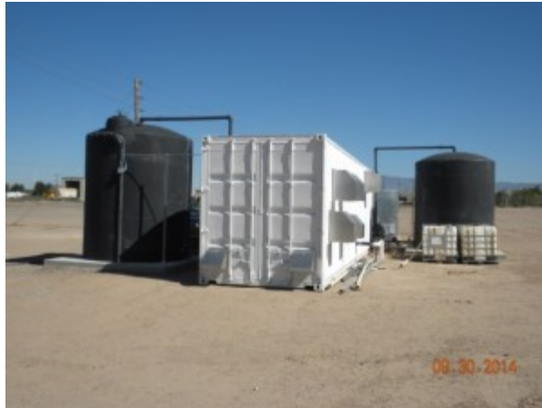
The nitrate plume treatment system compound where a soybean product amendment is injected into groundwater to breakdown nitrate in the contaminated plume.
