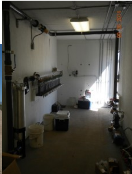
The nitrate plume treatment system compound where a soybean product amendment is injected into groundwater to breakdown nitrate in the contaminated plume.
