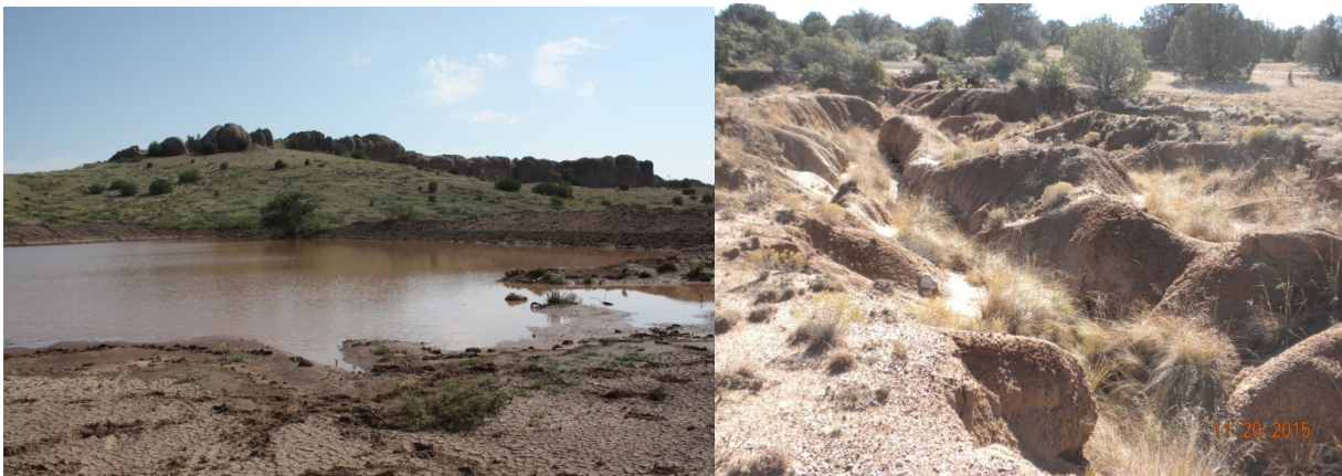
Examples of a surface stock tank (left photo) and an erosional gully created by run-off (right photo). Regrading and construction of berms for the stock tanks and the construction of erosional earthen structures for the gullies are among some of the restoration activities being implemented for this project.
