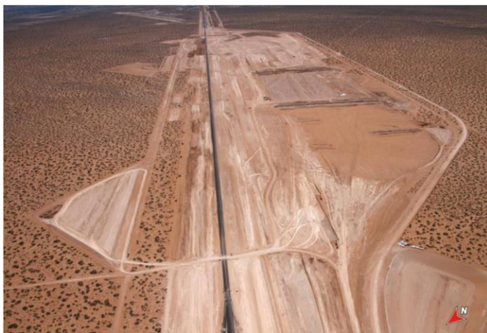
Santa Teresa grading work, May 2012.
