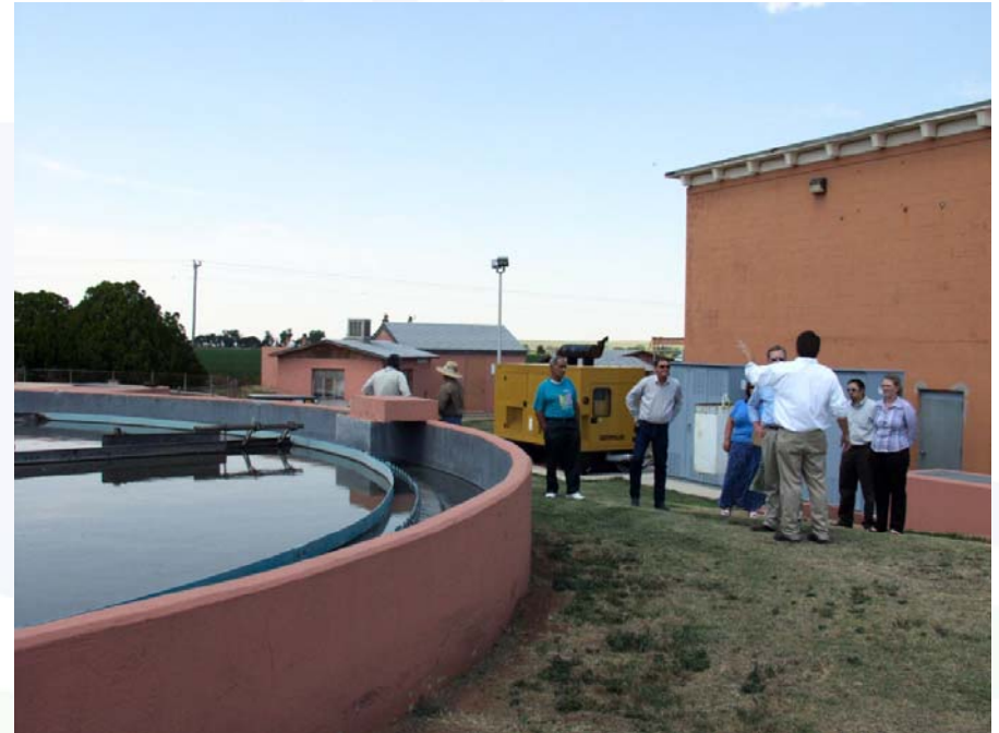
Tucumcari Wastewater plant. Rural Development assisted with the upgrade and modernization of the facility.
