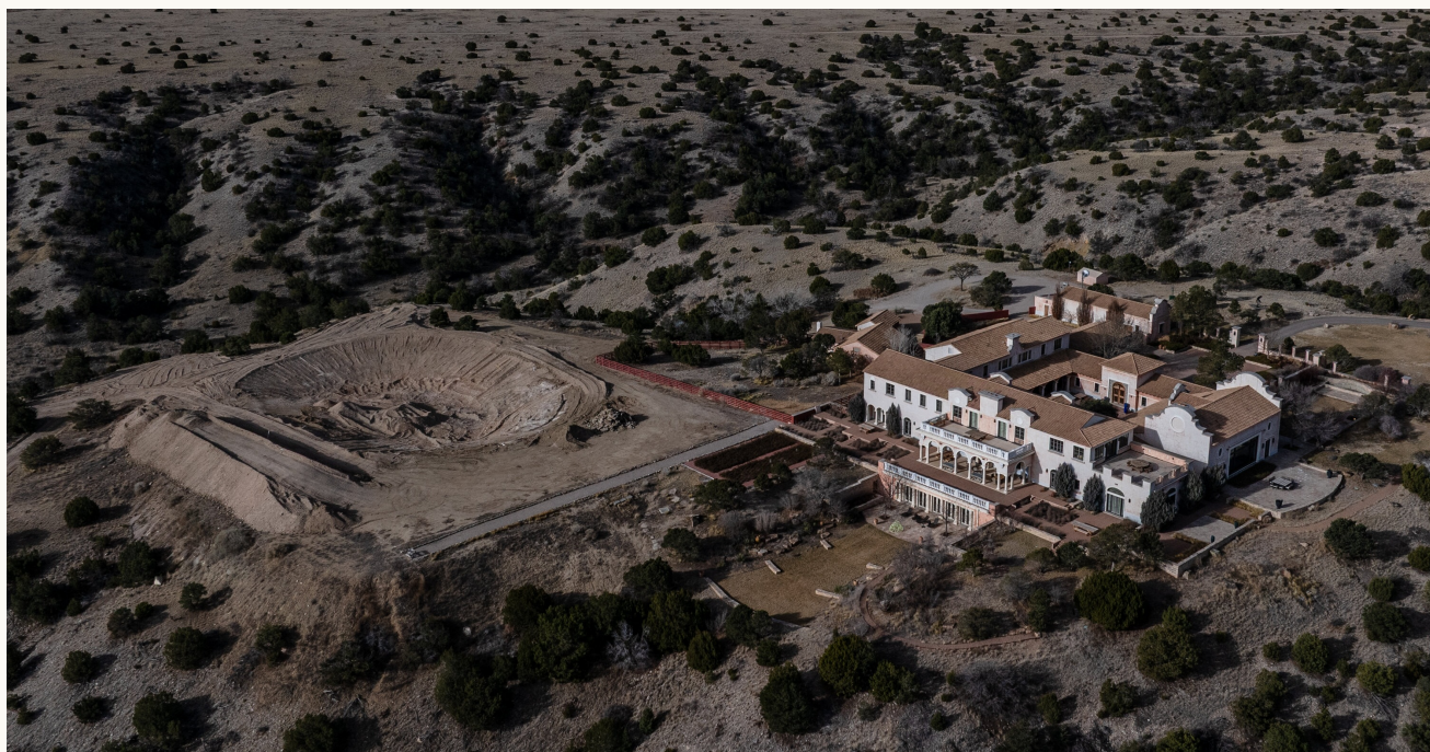
The main residence and outbuildings at the former Zorro Ranch, Stanley, New Mexico.
