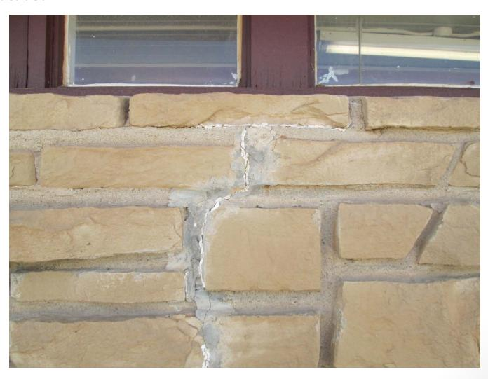
SASI Dormitory - Moisture from outside cracked walls to the interior wall. Cracks filled from outside as moisture barrier. Updated photo 09/18/13.
