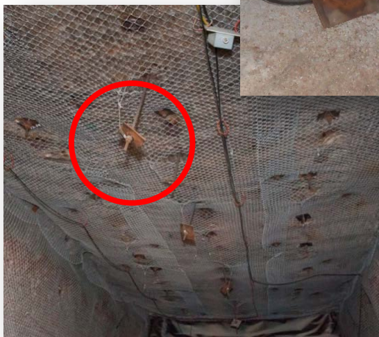
Broken roof bolts
