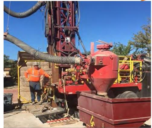
Using ARCH drill groundwater monitoring well
