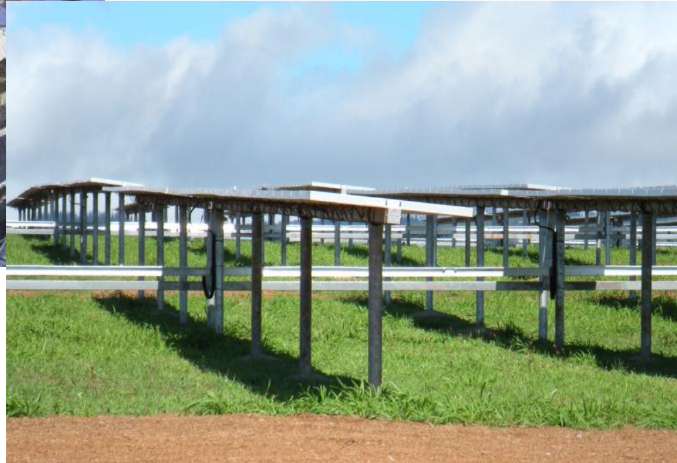
Lanai, Hawaii: 1.2 MW PV system on 4.5 MW island grid supplied by old diesel generators
