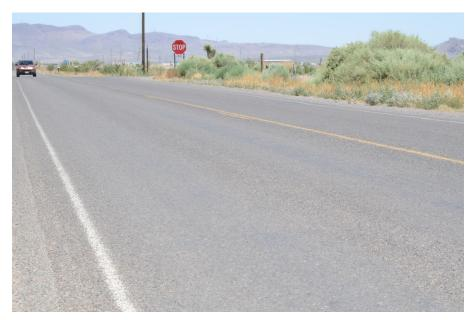
At left, Rockhound Road, which is part of the existing commercial truck bypass, is an example of the standards to which the Luna County Road Department would like to build new projects. Finished in 2015, it is rated for 80,000 pounds.
