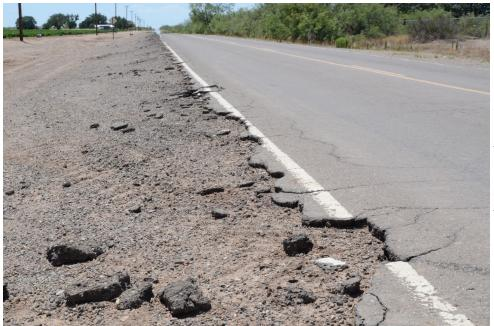
Solana Road is a former state highway and is approximately 6 miles long. Its travel lanes are 9 feet wide, instead of the recommended 10.5 feet. It sees heavy agricultural use, with tractor and semi tires causing shoulder damage
