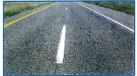
I-40 Crack Seal Project San Jon to TX State Line
