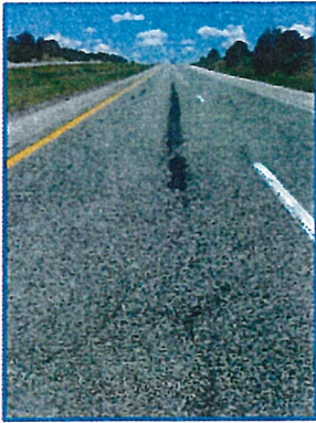
I-25 Plant Mix Wearing Course Project North of Rowe/Pecos
