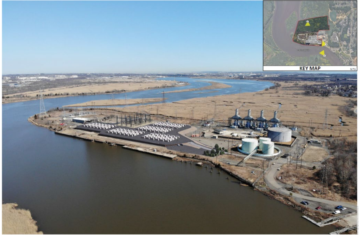
WOODS LANDING STORAGE
