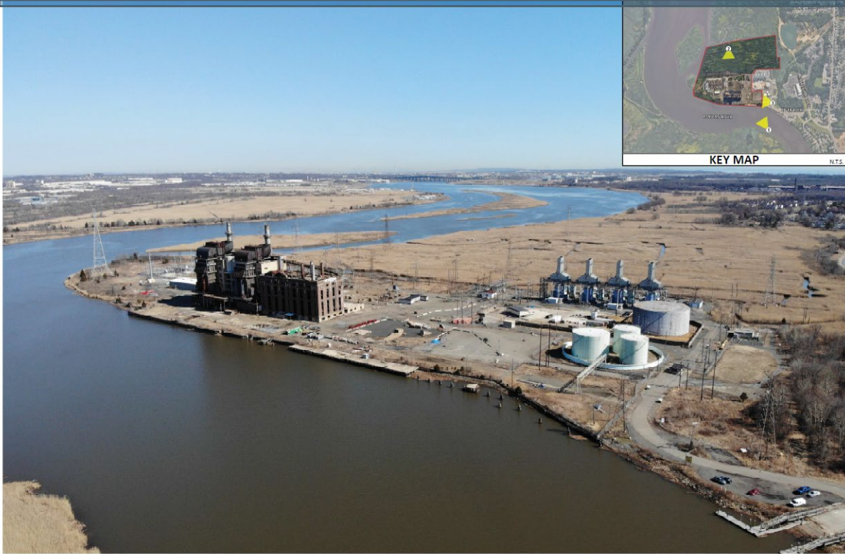
WOODS LANDING STORAGE
