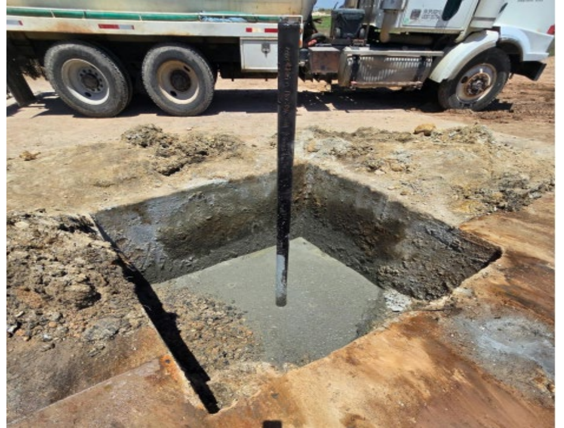
Post plugging, dry hole marker set
