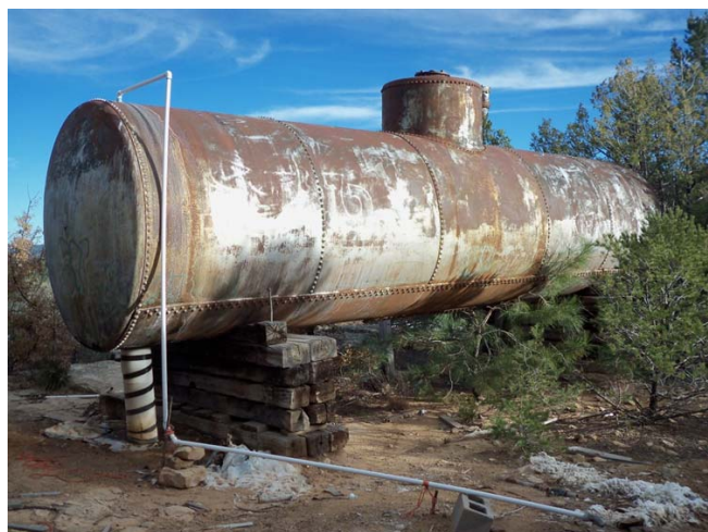
Greater Glorieta Regional Project Phase #2 Tank to be Replaced Funded by CO SAP
