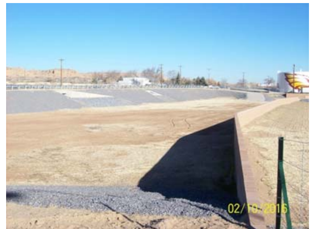
Completed Box Culvert in the Background
