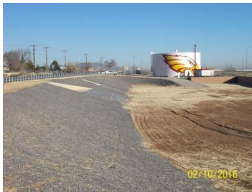
Completed North Pond
