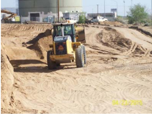
Excavation of North Pond
