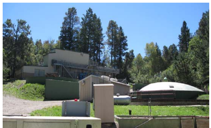
Cloudcroft Wastewater Treatment Facility Funded by RIP
