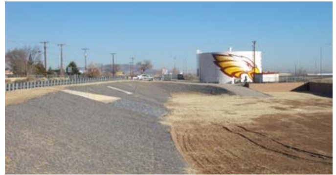
City of Belen Drainage Pond Funded by CWSRF Program
