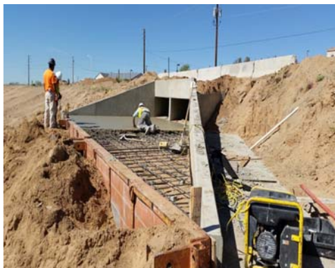
Concrete Box Culvert that Discharges to the North Pond
