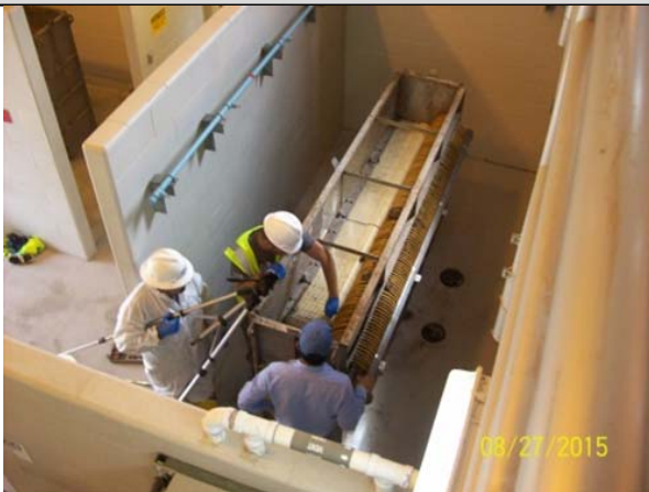
Existing MBR cassettes being cleaned and inspected prior to re-installation
